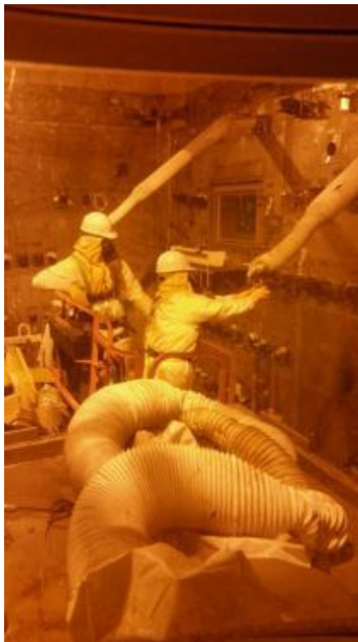
Vitrification Cell – Placing Manlift in Cell and Preparing Manipulators for Removal
