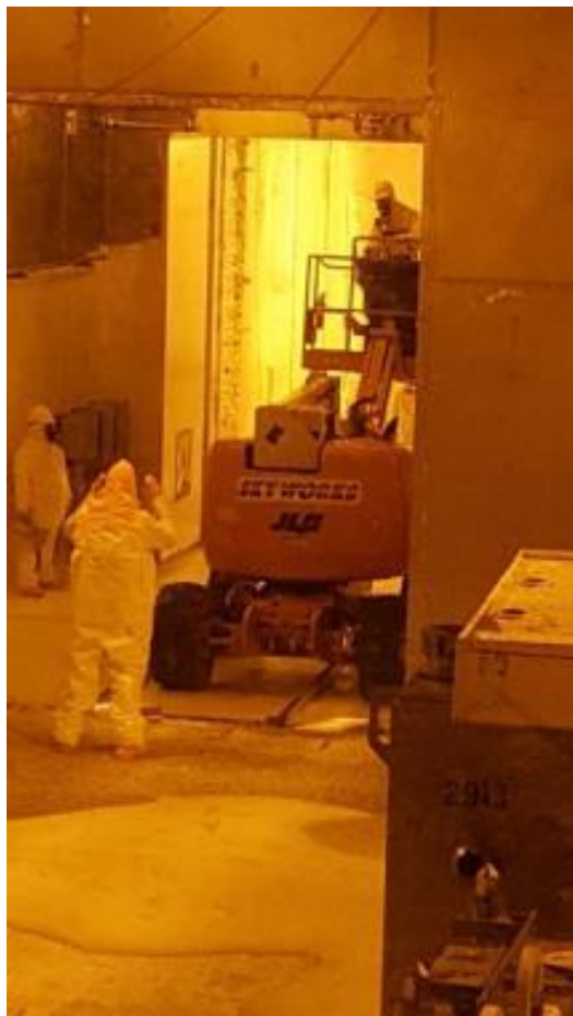
Vitrification Cell – Placing Manlift in Cell and Preparing Manipulators for Removal
